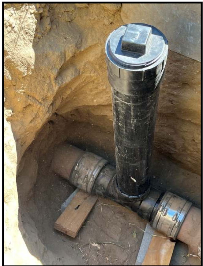
Installed a sewer clean out on Hayes Dr.
