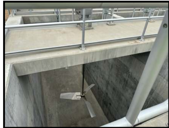
Figure 4: Floc Basin – Flocculation Chamber
