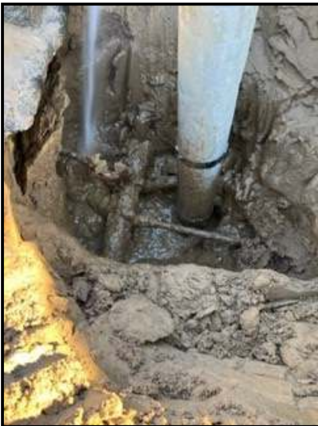
Repaired water leak on S. Laurel St.
