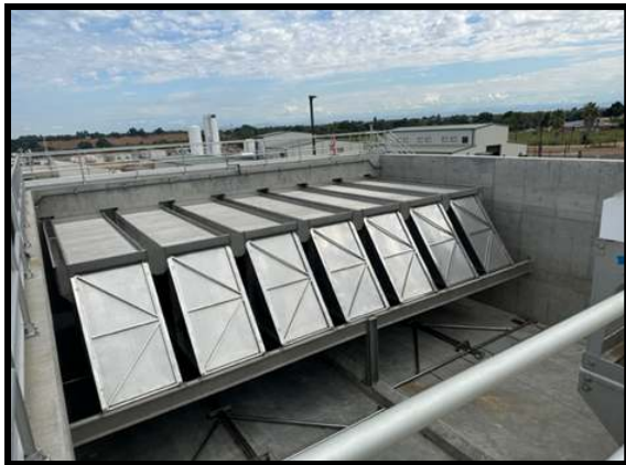
Figure 3: Sedimentation Basin – Plate Settlers
